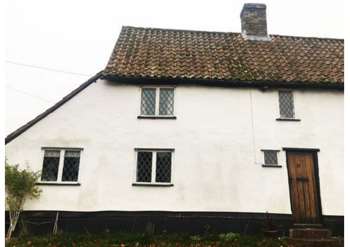
Fig 17 Rendered Church End cottage with black pitch plinth and catslide pantile roof
