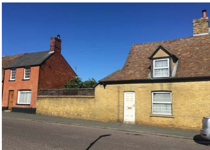
Fig 61 Church Street, Variation in form of clay and slate roofs including dormers and hips.
