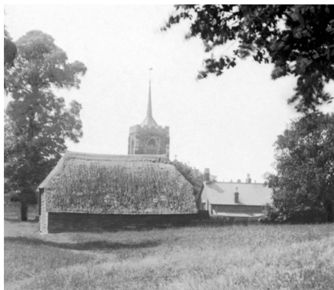
Fig 60 Former Tythe barn near the church, demolished
